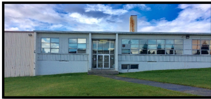
HERC-1 Upper Level Entrance
