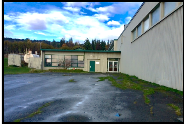
HERC-1 Lower Entrance Used to Access Gymnasium
